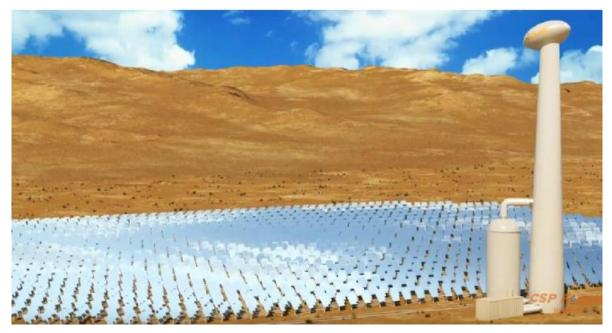
Most heliostats are usually stowed at night with their mirrors facing the sky. This can cause the mirrors to be soiled by a sticky mix of moisture (dew), dust, and air pollution. They also are subject to adverse weather, including sandstorms and hail. In much of the Middle East, for example, great expense usually is required to clean the hard-to-remove dirt from the mirrors that's been deposited at night.
